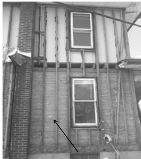
Exterior siding removed
